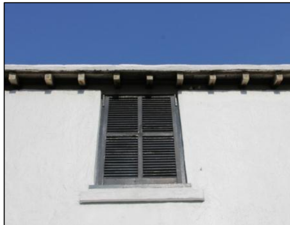
Stewart Hall in St George's has had a wooden roof/wall plate for almost 300 years
