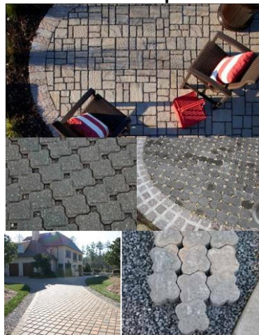
3. Permeable interlocking concrete pavements
